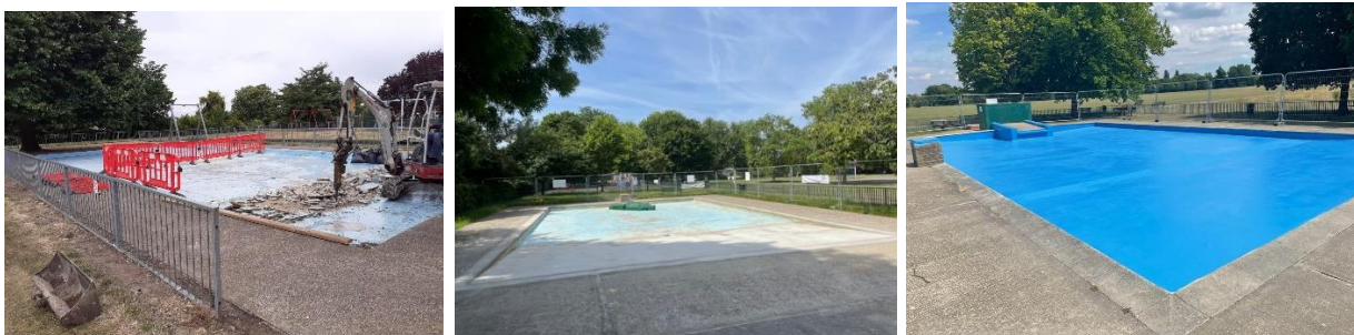
DDA 1:12 access ramps to all 6no Paddling Pools in Merton Parks June 2022
